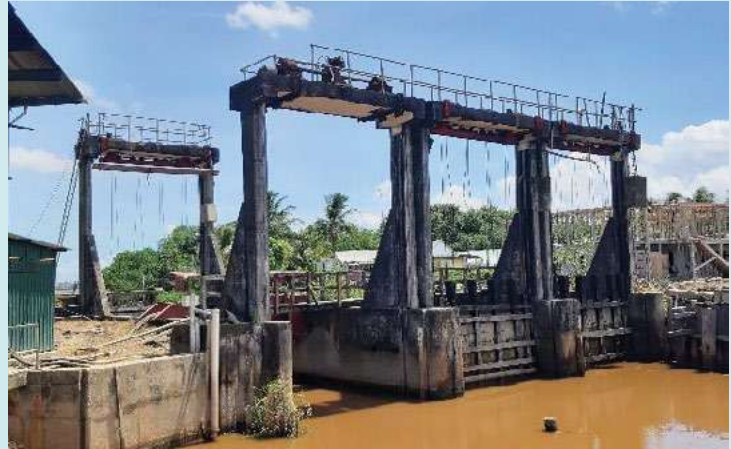
Canal No.1 Sluice – West Demerara, Region 3
