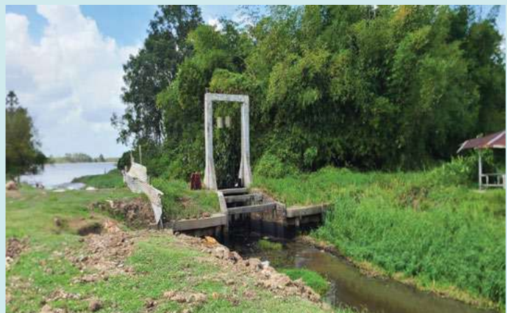
Garden of Eden (GDF) Sluice – East Bank Demerara, Region 4
