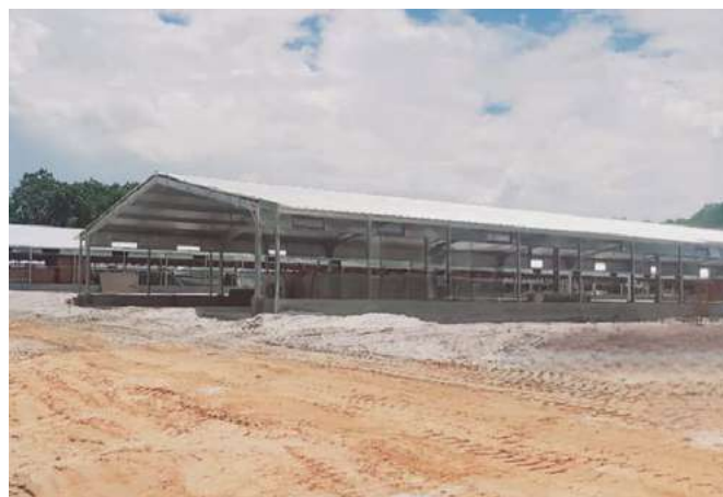
Tunnel House under construction at Bounty Farm Ltd.
