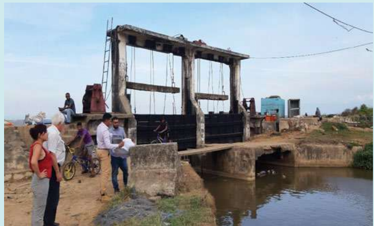
Greenfield Sluice – East Coast Demerara, Region 4
